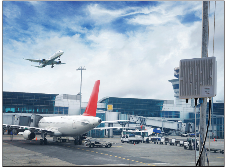
Fig 8. Anritsu Remote Spectrum Monitor Positioned at Airport
